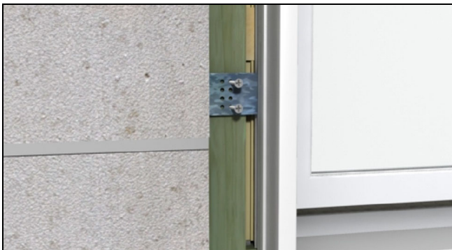
Figure 19 Attaching window with structural brackets.
