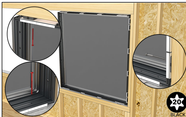
Figure 23 First unit (A1) when mulling in an opening.
