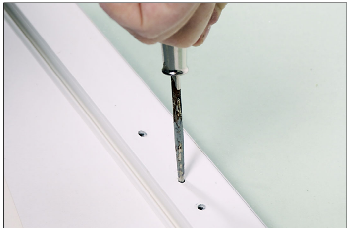
Figure 4: Use scratch awl to move backer.
