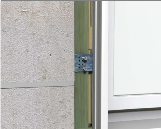
Figure 17 Attaching window with structural brackets.
