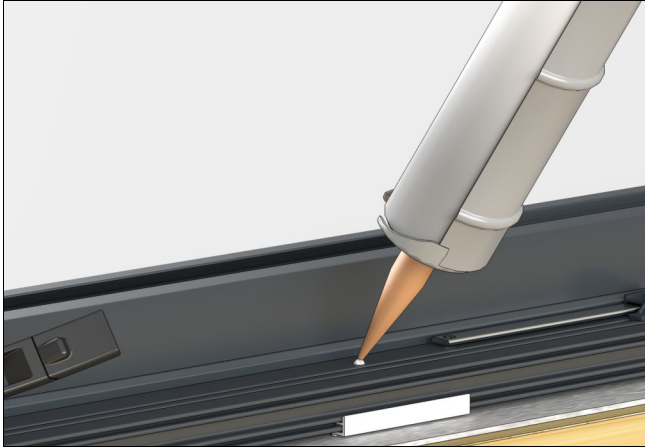
Figure 32 inject installation holes with sealant prior to fastening.
